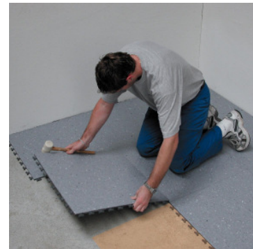
Once the first two rows are complete, the entire area can be gradually laid.
