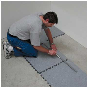
Mark out the cutting edge and cut with circular saw or jigsaw.
